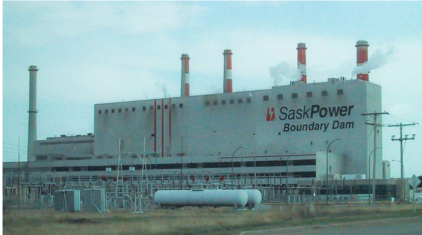
Sask Power - Carbon Capture
